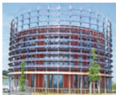
Office of Energy Syndicate of Drôme department (14 kW, photo courtesy Tenesol).
