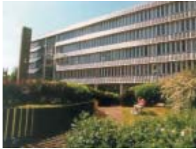
▲ Figure 6.3: University of Northumbria, UK. This 39.5 kWp installation is the result of a refurbishment project at the University of Northumbria in Newcastle. Photovoltaic panels have been incorporated into the new over-cladding of the building and the electricity produced contributes to meeting the building's needs for lighting, computers and other appliances. Any surplus electricity can be fed into the University's internal distribution system to supply other buildings on the campus. Source: Tymandra Bewett-Silcock.
