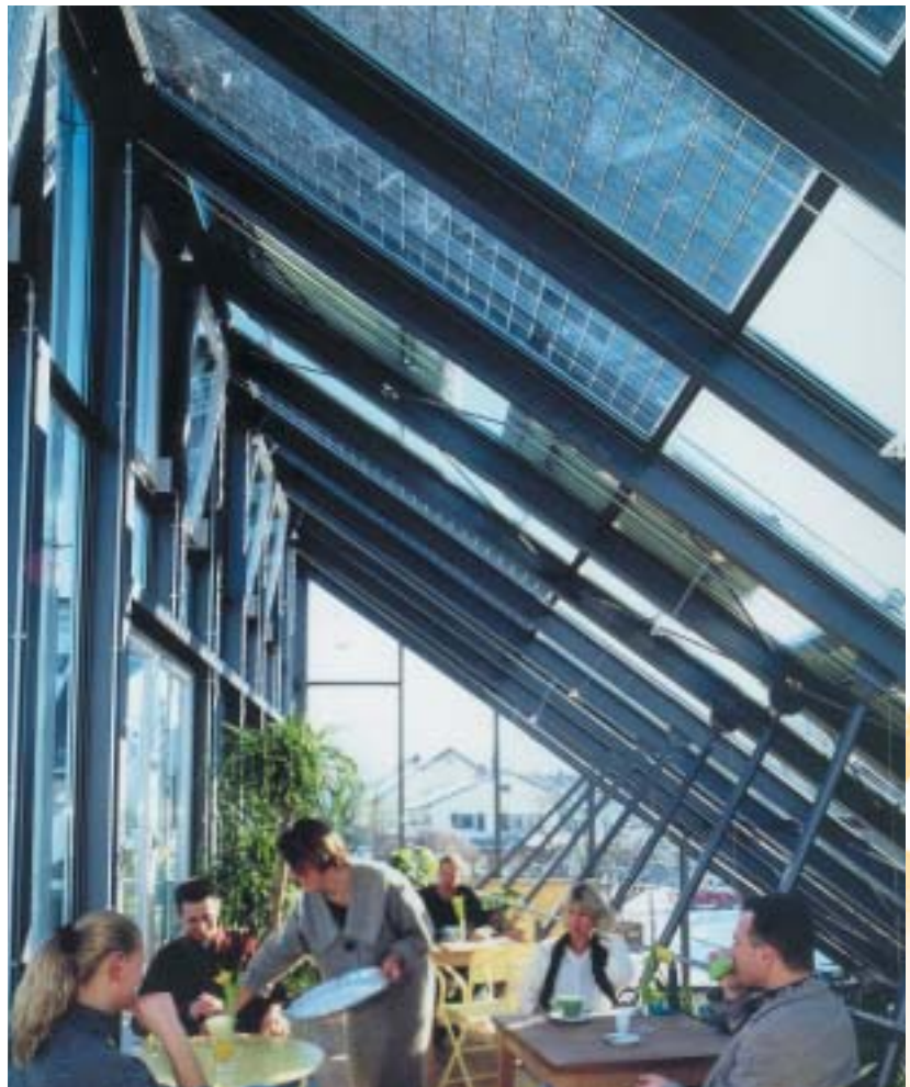
▲ Figure 1.3: Intelligent building design and construction process - mounting and integration of solar modules into the Mataró library building in Barcelona, Spain. The photovoltaic modules are at the same time façade elements and are part of the solar power station (53 kWp). Source: TFM, Spain.
