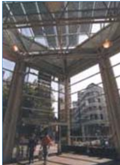
◀ Figure 7.9: Migros Limmatplatz Solar Power Station in Zurich, Switzerland. Installed capacity: 30 kWp. Energy production: 24000 kWh/yr. Photovoltaics surface: 360 m 2 . Investment cost: 190000 €. Financing: Solar Stock Exchange. Source: energiebüro®, Zurich, Switzerland.
