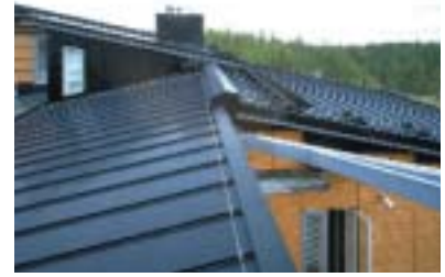
▲ Figure 6.10: Flexible roofing laminates for membrane roofing are available on the market. Source: Uni-Solar - Bekaert ECD Solar Systems LLC, Belgium.
