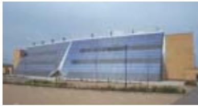
◀ Figure 5.12: The Doxford office building in the UK shows the integration of photovoltaics in a contemporary setting of a business park. Source: Studio E. Architects, London, UK.
