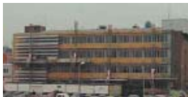
▲ Figure 5.14a+b: Before (a) and after (b) refurbishment and integration of photovoltaic modules to façade as shading devices (building in Petten, NL) Source: http://www.pz.nl/bear/bearecn8.html (Thermie project SE 100/97/NL/DK - photovoltaic projects).
