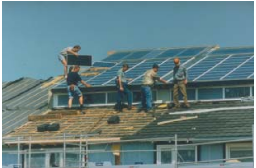
▲ Figure 0.2: Roof to be clad and turned into a multifunctional building skin. Source: Ecofys, The Netherlands.
