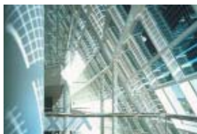
◀ Figure 5.4 a+b: Photovoltaics incorporated as shading elements – building for the University of Erlangen, Germany (a) vs. semi-transparent photovoltaics – Doxford office building, UK (b). Source: (a) Solon AG, Berlin, Germany. (b) Studio E. Architects, London, UK.
