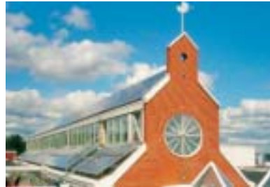
◀ Figure 5.13b: Combining photovoltaic integration and respect for traditional building styles in new construction is possible as this example clearly shows. (Lieliahti Citymarket in Tampere, Southern Finland), Source: Naps Systems Oy.
