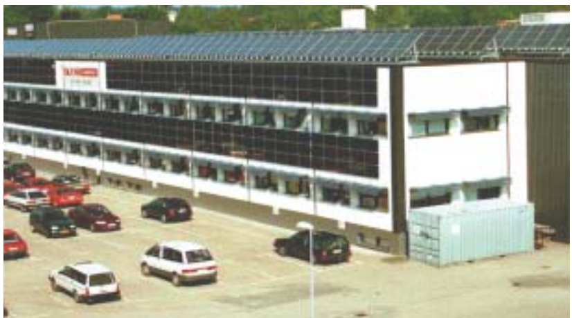
▲ Figure 7.5: IKEA offices, 60kWp roof and façade. Source: Energibanken, Jättendal, Sweden.
