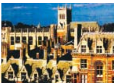
▲ Figure 5.11: Listed buildings and conservation areas present a challenge for BIPV potential (Cambridge, UK).
