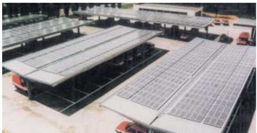
▲ Figure 1.7: Car shelter and photovoltaic power station in one. Source: Anit, Italy.
