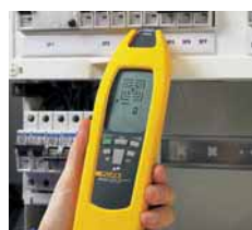
Location of fuses/breakers and assignment to circuits
